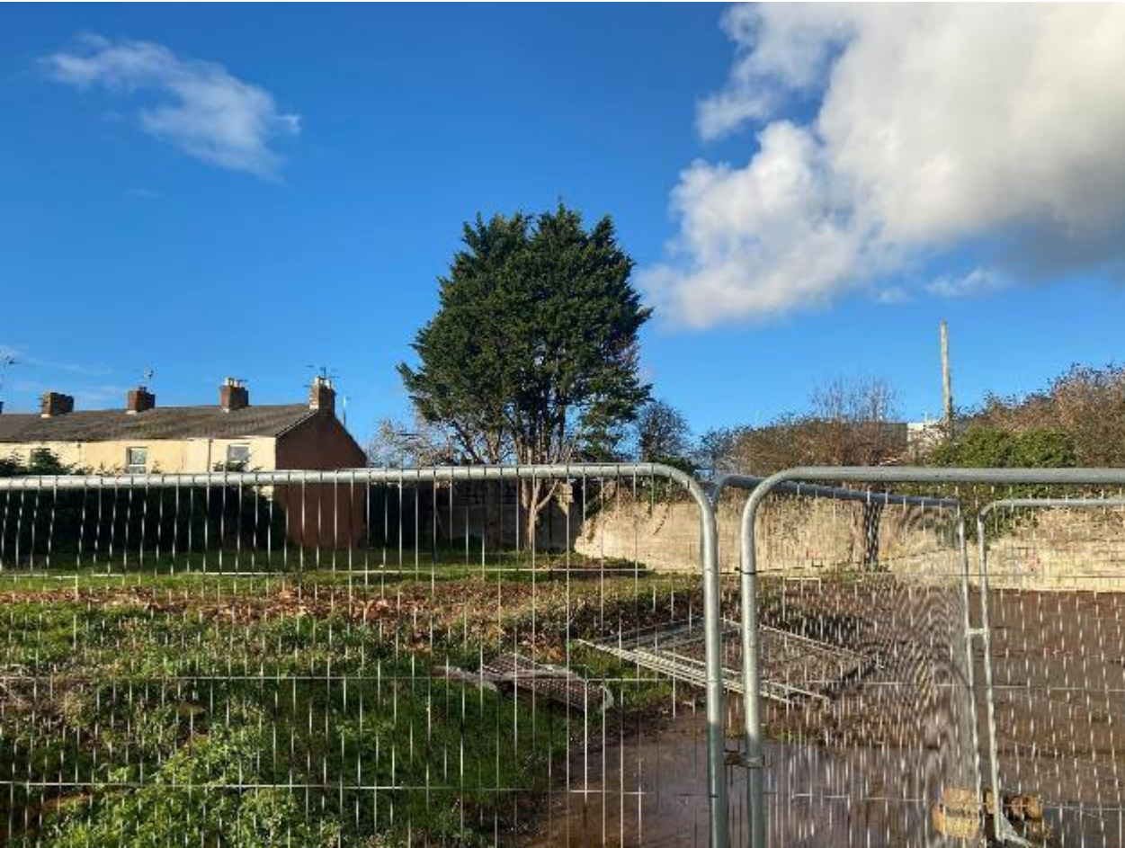
View looking north across site
