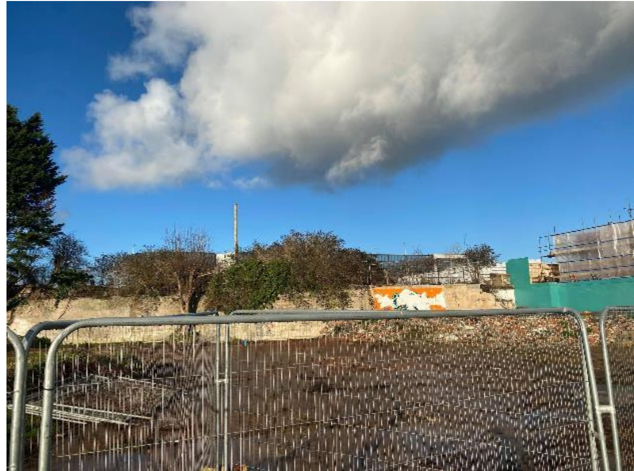
View looking north across site
