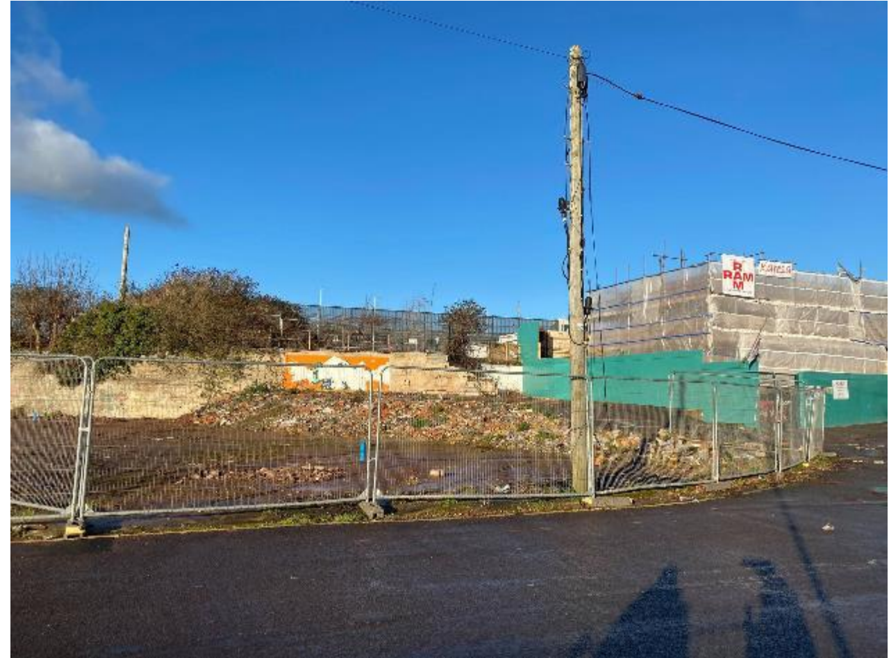
Eastern portion of proposed site. Old railway building covered in scaffolding
